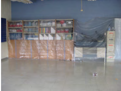
Ready for lighting demolition
