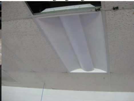
New Lighting Fixture
