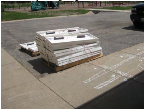
Light Fixtures that were removed
